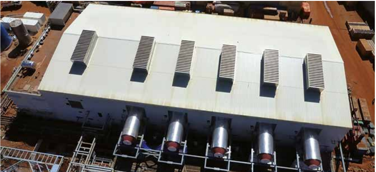
Thika Power Plant - Kenya / Taşyünü Cephe Paneli
